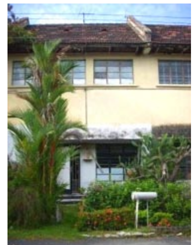
There are only three units left still with occupants. The rest have left to make way for the demolition job. This is the front view of Ms Rosy Tan's residence.
